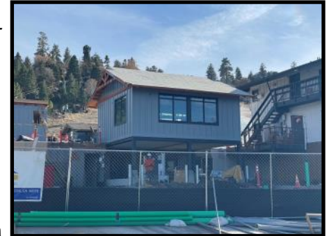
A view from the parking lot of the new USARC building
